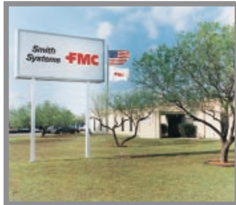
The Smith Systems Operation facility, located in Corpus Christi, Texas, has strategic access to the petroleum industry and the city's international deepwater port.
