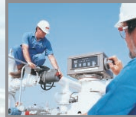
Smith personnel oversee every aspect of system design, fabrication, and commissioning to ensure flawless operation.
