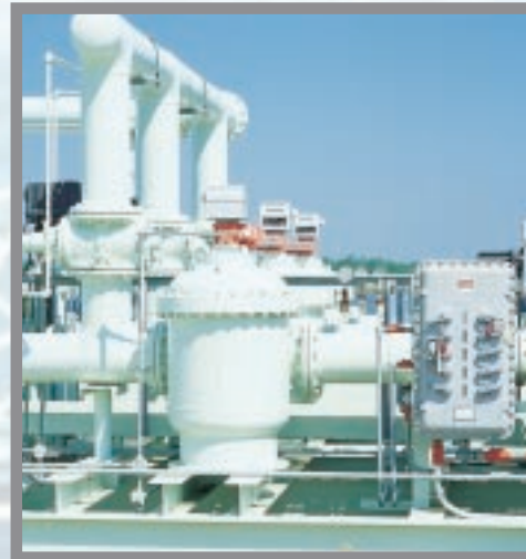
PD meters ensure accurate, reliable, custody transfer measurement in marine loading applications.
