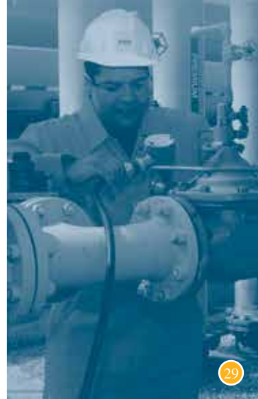
4" Unloading Skid with Model AR Air Eliminator
