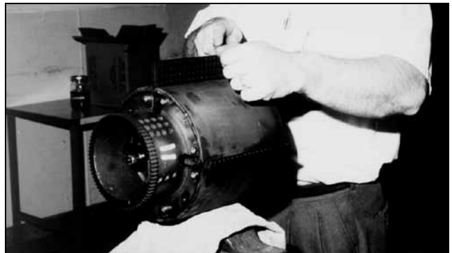
Figure 21 – File Blade to Increase Blade Tip Clearance
